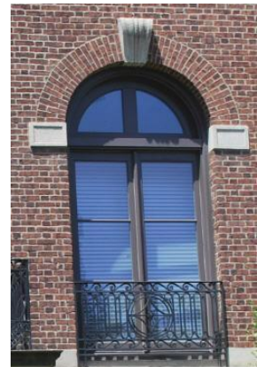
Figure 2: Romanesque arched windows
